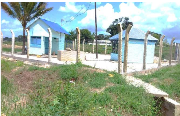
Pump and pressure vessel houses at Ole Scheme
