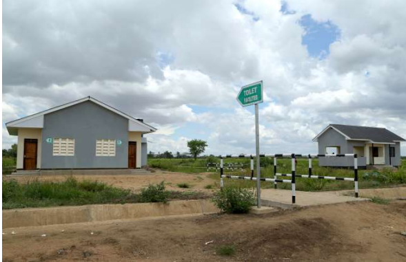
Resting shed and toilets at Mvumi Irrigation Scheme, Kilosa
